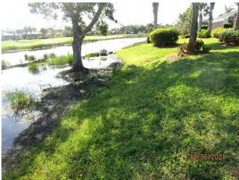
Shoreline between Lakes 3 & 5 Washout at 9129 & 9131 Shadow Glen
