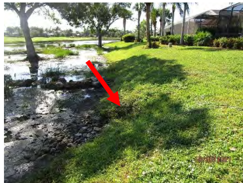
Shoreline between Lakes 3 & 5 Washout at 9129 & 9131 Shadow Glen
